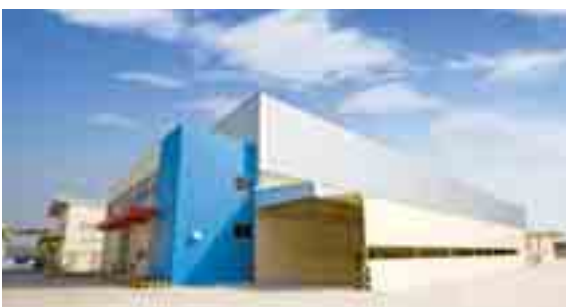
Otsuka Pharmaceutical Storage Warehouse Samuthsakorn, Thailand | 2011
