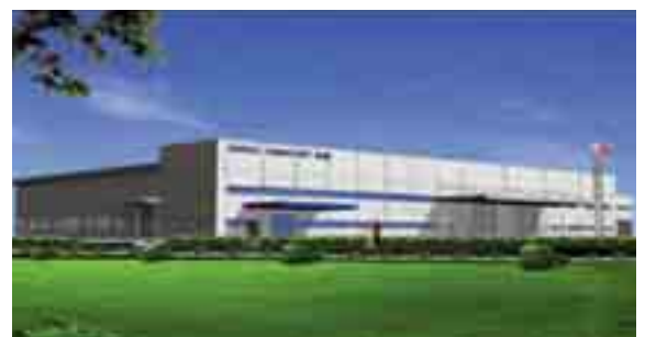
Enshu-Sanko Vietnam Factory Bac Ninh Industrial Estate, Vietnam | 2012
